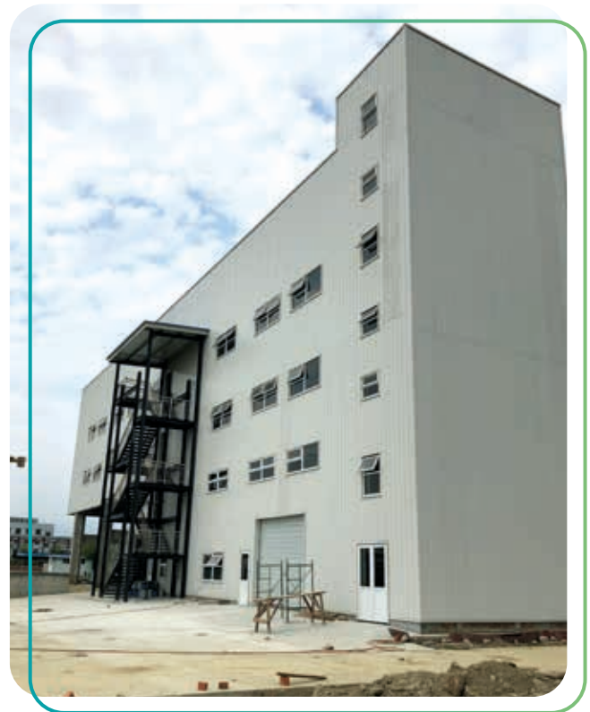
Facility at Jiangyou (江油设施)
