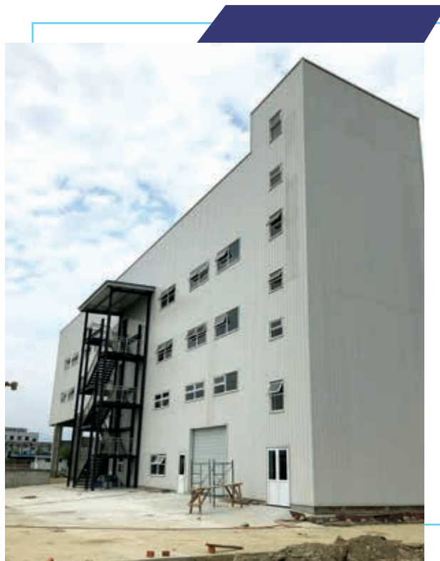
Facility at Jiangyou (江油设施)
