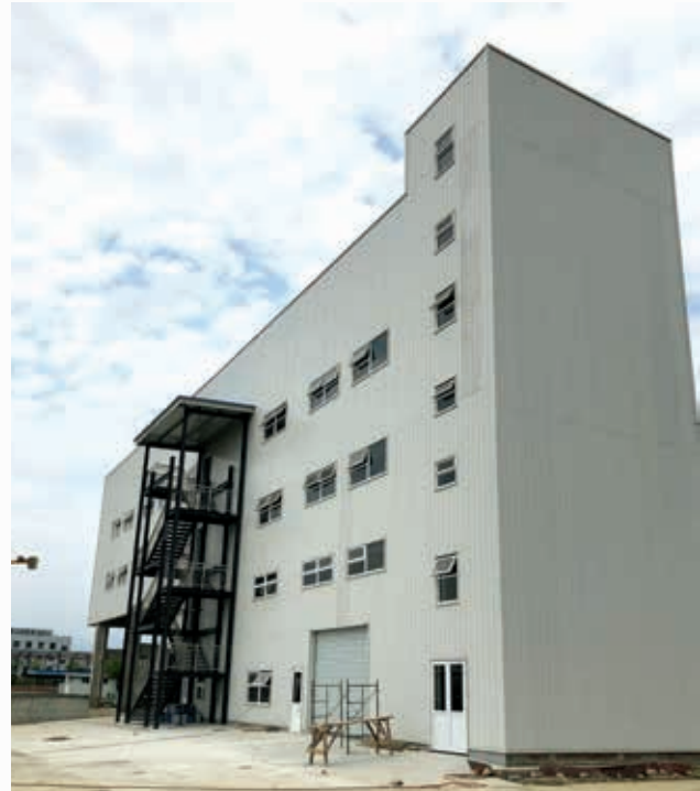
Facility at Jiangyou (江油设施)
